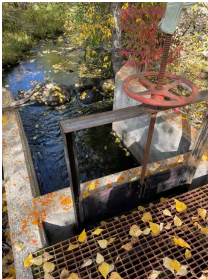
Slide Gate and Section of Downstream Channel
