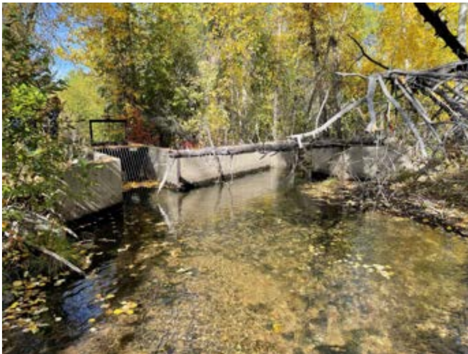
Upstream Side of Diversion Channel, Bar Screen, and Slide Gate
