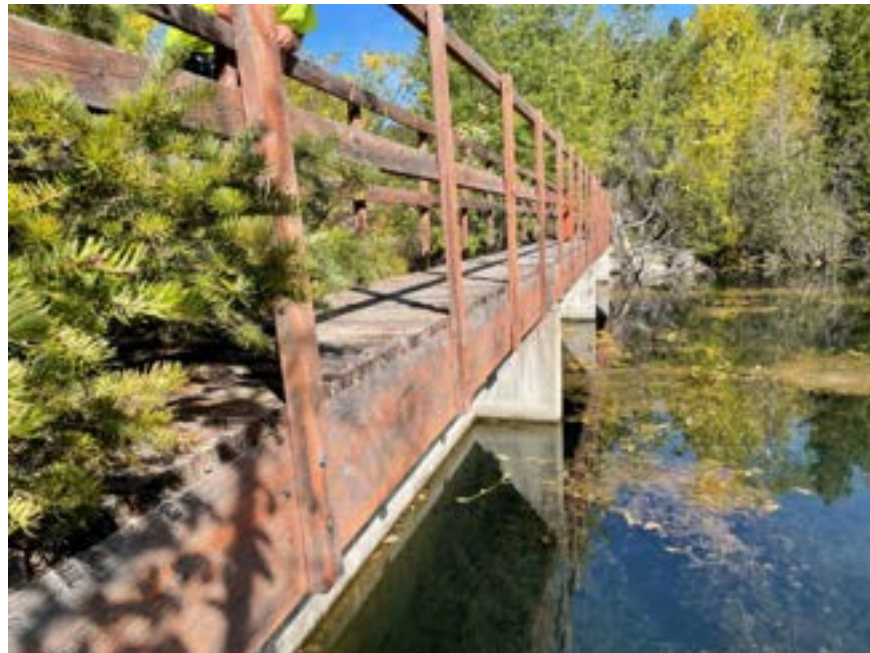
Upstream Side of Dam showing Catwalk, Orange-Colored Pedestal, and Pond
