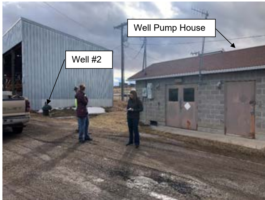
Existing Well Pump House showing Well #2 Location outside of Pump House
