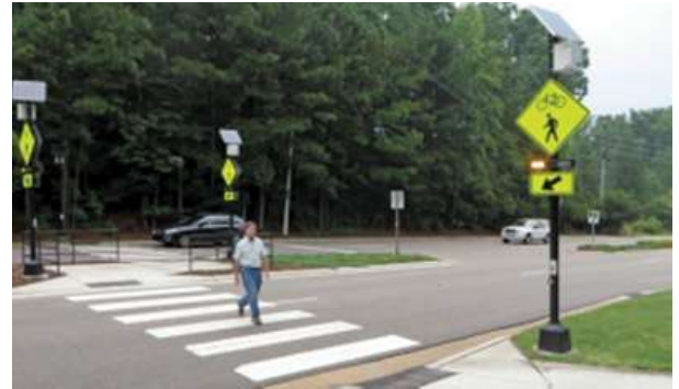
▼ Figure 8 - Crosswalk with Pedestrian Flashers
