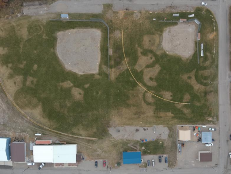
Figure 2 - Springs Park Drone Photo
