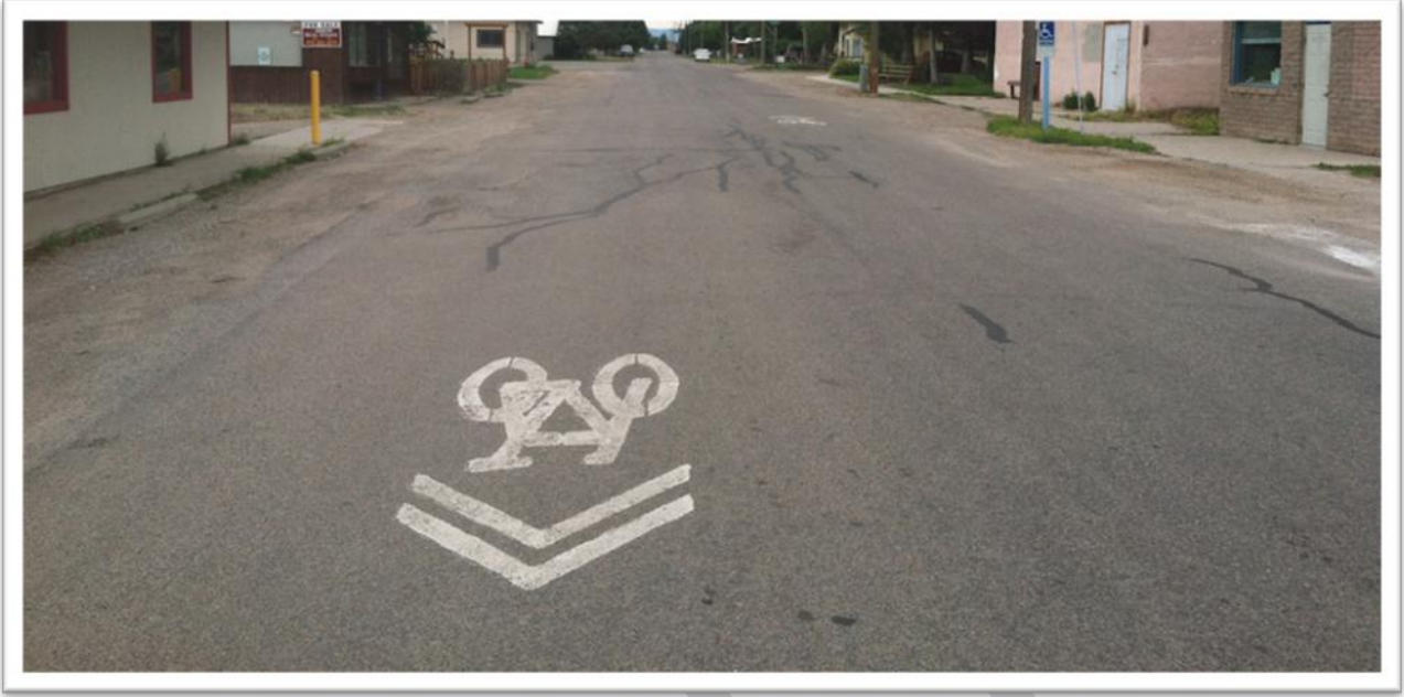
Figure 9 - Sharrows in Ennis, MT. Source: Federal Highway Administration 'Small Town and Rural Design Guide'
