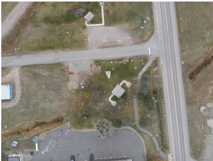
Figure 7 - Radar Park Drone Photo
